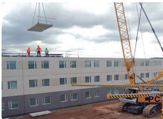
Lifting precast slabs into position.
