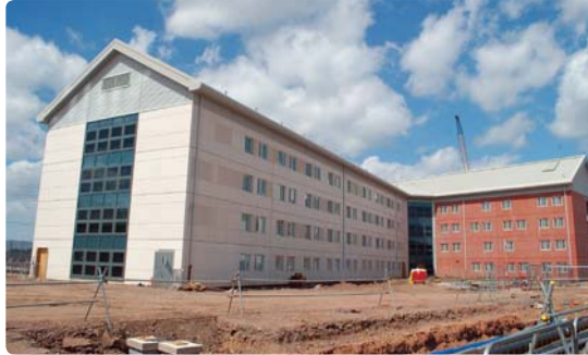
The terracotta façades on house block entrances have been used to aid site co-ordination for prison staff.
